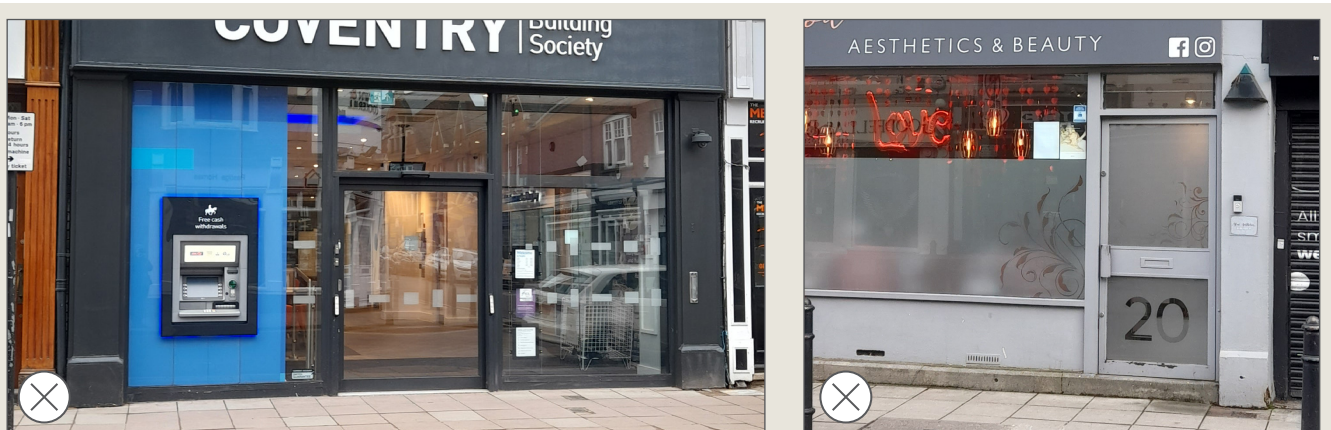
Left and right: These shopfronts have lost their historic entrances and present a flat presence to the street with no depth to the entrance sequence. They have also lost any original materials or details as a result.
