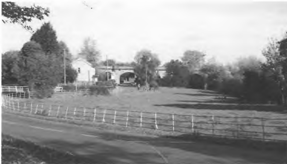
The railway bridge carrying the west coast main line from London to Birmingham.
