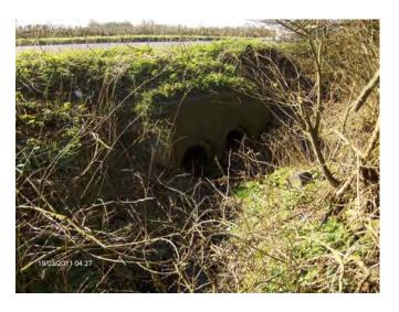
Partly silted culverts under A45
