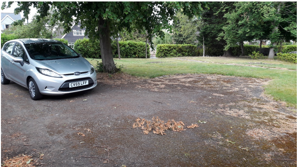
Existing driveway layout. Minor debris (twigs and seeds) on driveway
