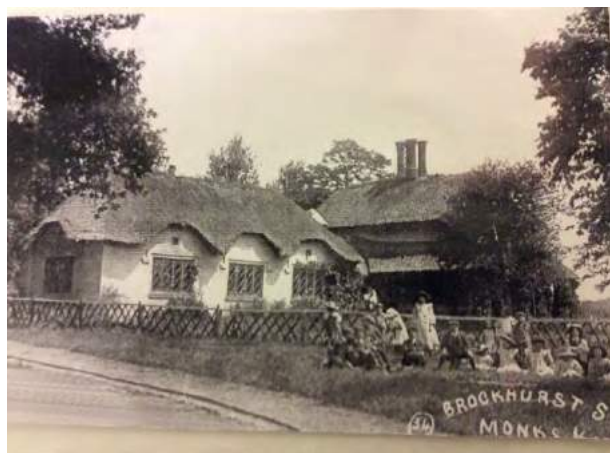
Brockhurst School pre-1912
